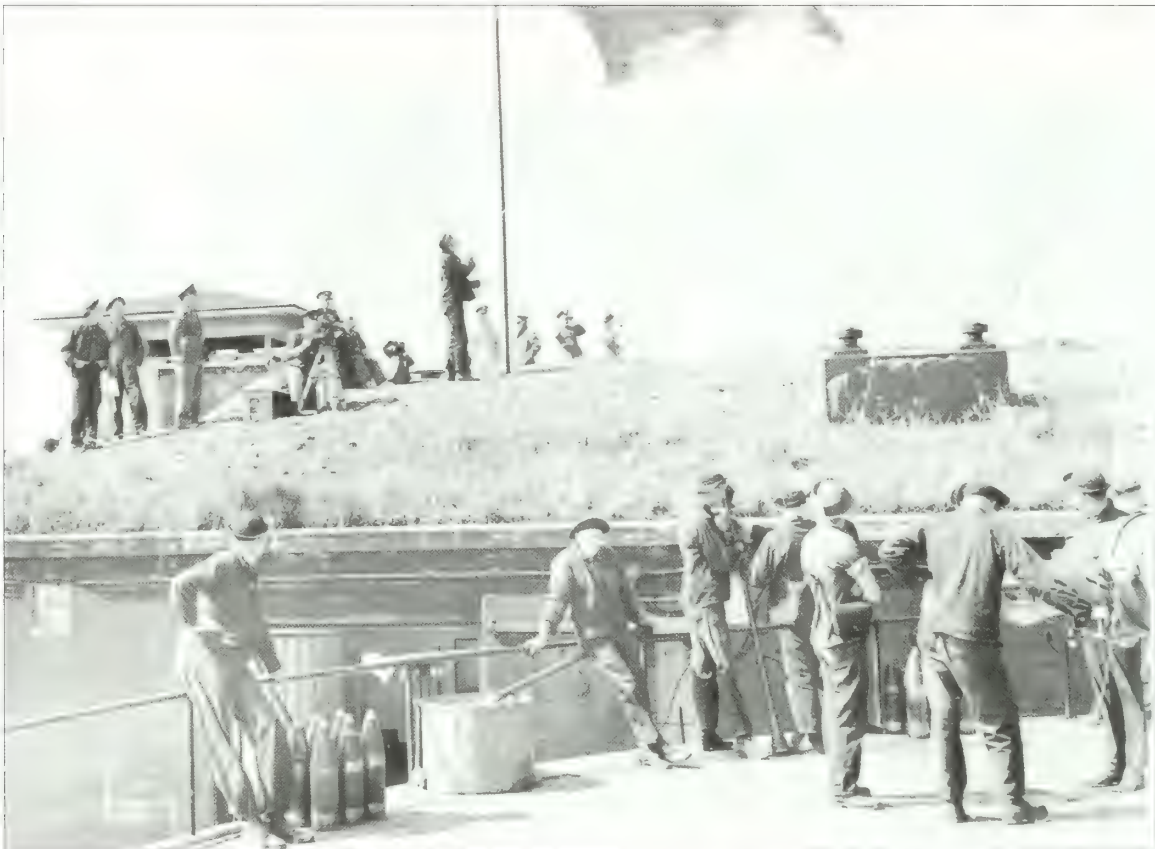
Figure 4.13. View looking north from emplacement #1 at commander's station, shell hoist, and central structure, Battery Gunnison, circa 1940. Soldiers are seen on top of the earthwork in front of the commander's station, however, the photograph does not reveal defined circulation routes. Today, visitors have formed a trail between the emplacements that also loops around the shell hoists and battery commander's station (GATE 13708).
